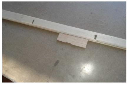
Taper the longerons at the rudder cutout so the back end of the fuse can be glued to the rudder.
